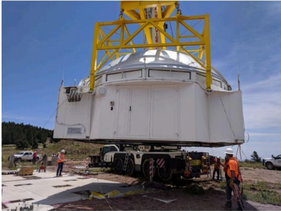
Figure 4: UT being installed on array pad.
