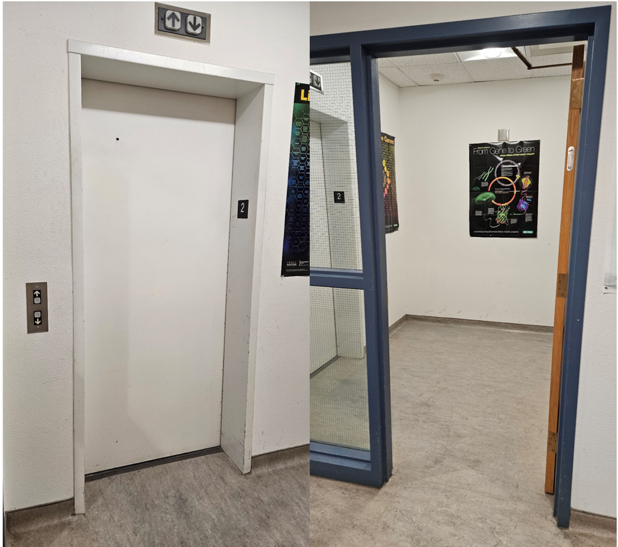
Figure 11. Elevator door access and doorway.
