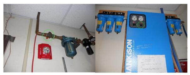
The gas is pictured on the left, turn the perpendicular red handle to the open position such that it is parallel with the pipe. On the right is the Blue Hankison unit, flip the rightmost switch to the on position. Order is crucial in this step to prevent damage to the instrument.
