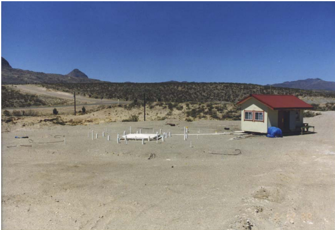
Figure 5: View of the test site looking west. Infiltrator, covered with white plastic sheeting, pictured in the center. Data loggers and supply tanks are housed in the small building to the north (Brainard et al. 2002, Baker 2001, Paprocki 2000).
