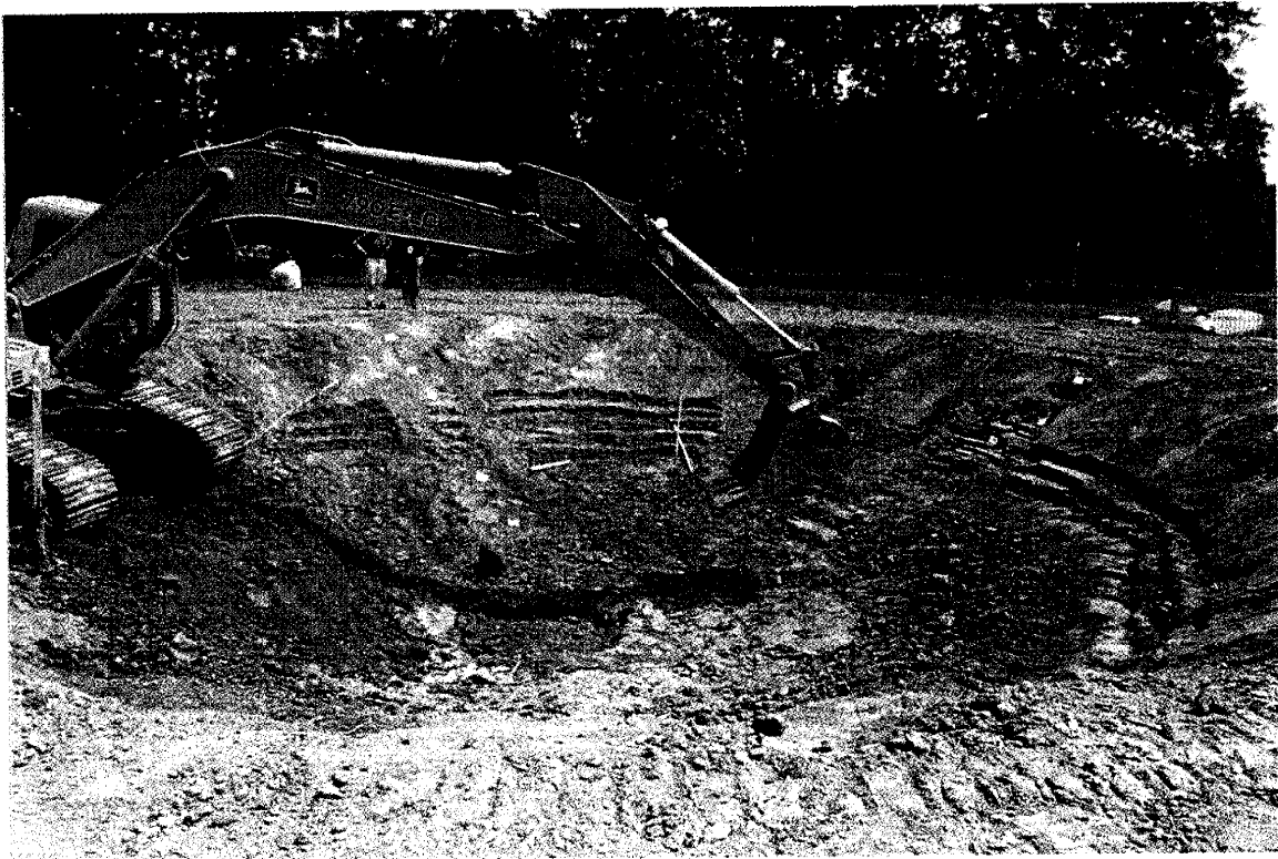
Plate 59. Back hoe excavation and sloping of sides. The blue tarp was put in place to prevent movement of the remnants of the dye pit.
