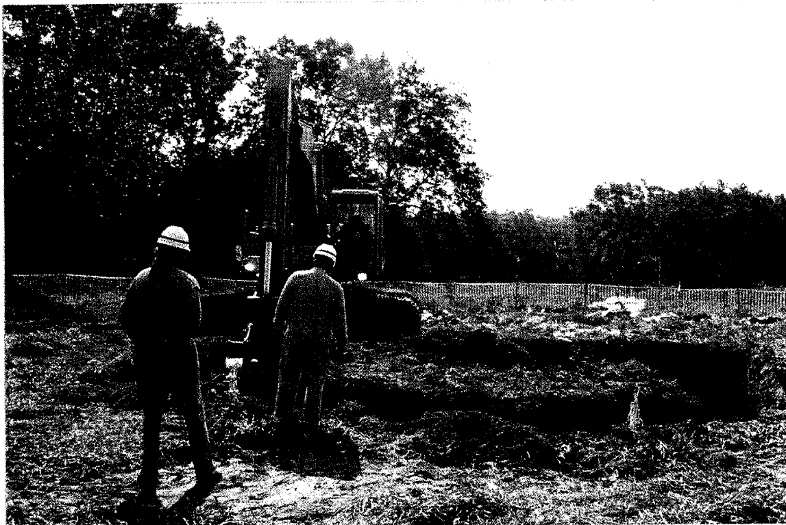
Plate 22. Back hoe trenching between inner and outer sampling rings.
