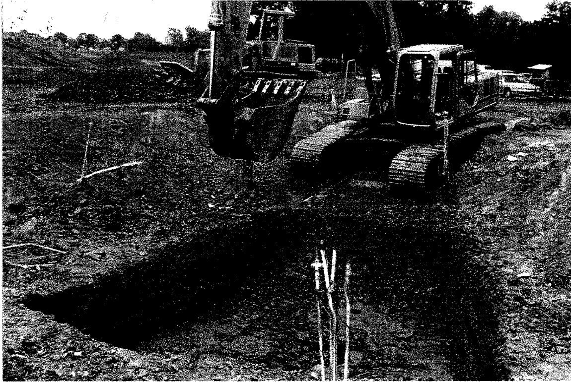
Plate 48. Deepening excavation to the top of Unit 2, layered unoxidized clays.
