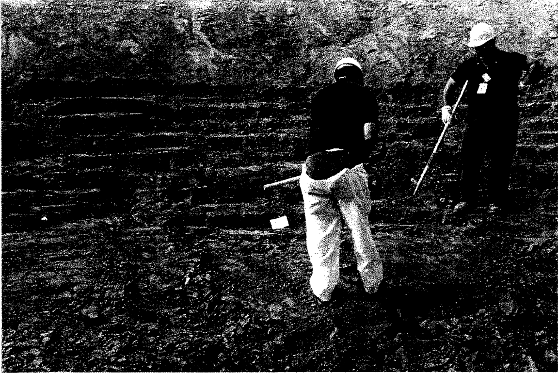
Plate 70. Hand terracing of sloped excavation sides.
