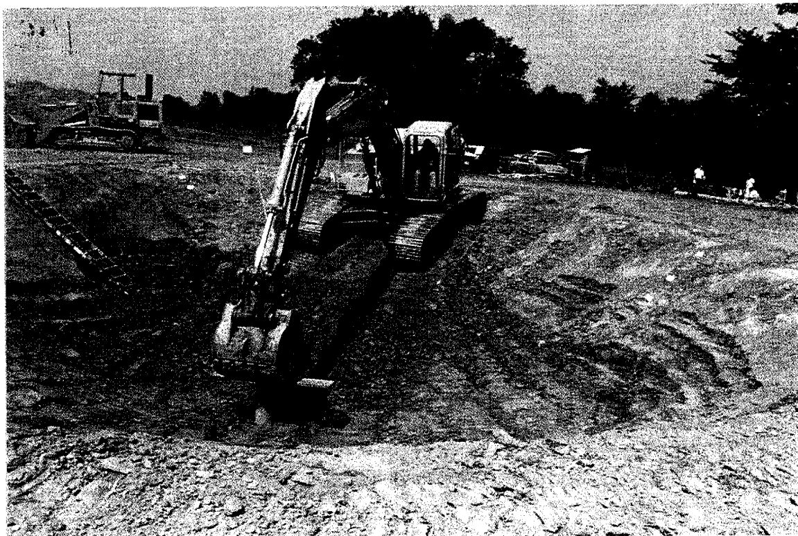
Plate 61. Back hoe used to press pipe into media for core samples.
