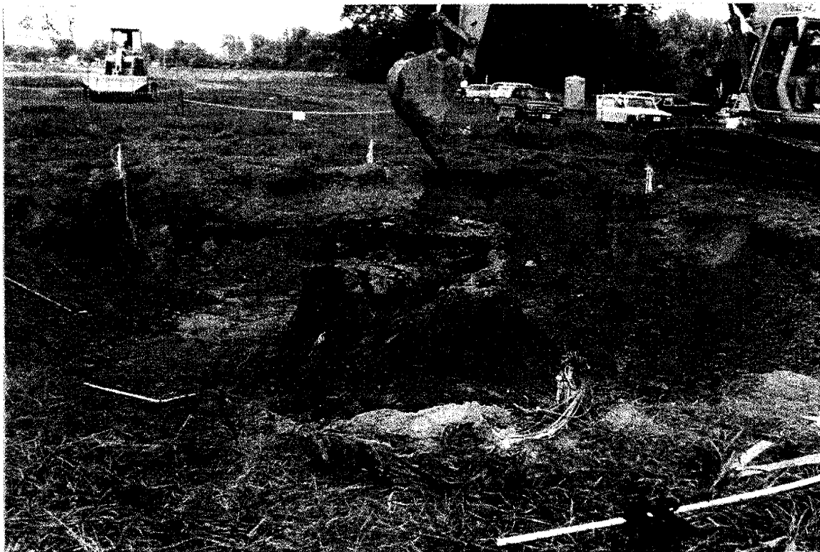
Plate 26 (below). Back hoe excavation between the infiltrometer and the outer sampling ring.
