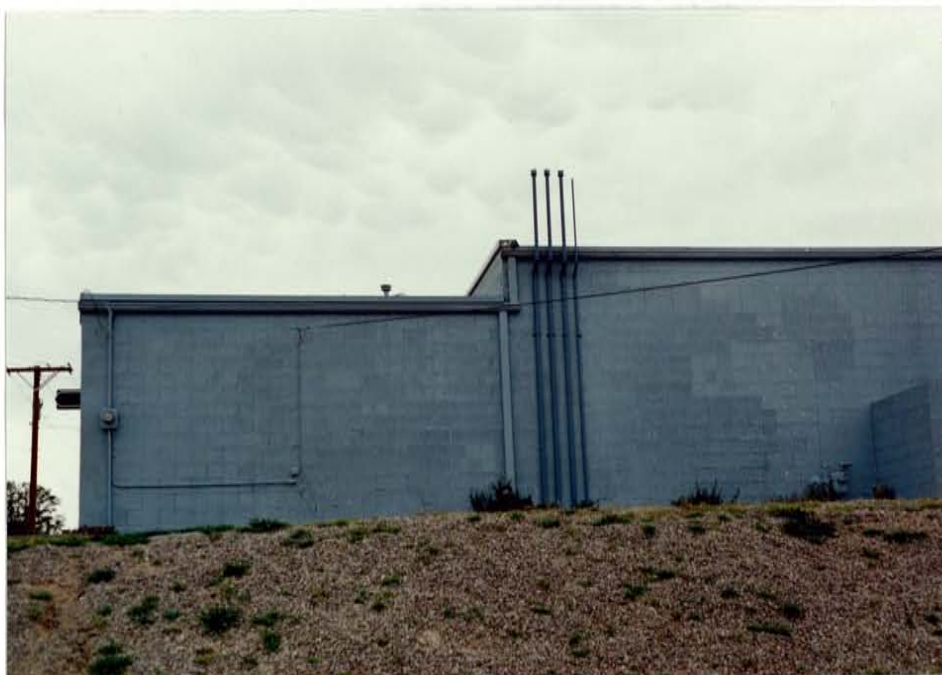
Figure 20 Photograph of UST vent pipes. Three larger pipes are vents for standard size USTs(1000-8000 gallons). Smaller pipe is most likely a vent for a smaller (<500 gallons) tank.
