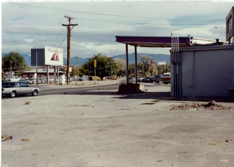
Figure 22 Photograph of deserted gasoline station. Notice the four vent pipes near the edge of the building and the numerous refill cap covers and manhole covers in the foreground of the picture.
