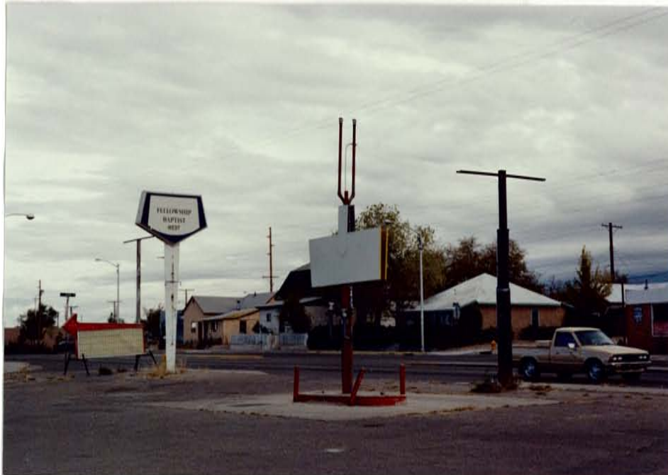
Figure 21 Photograph of abandoned gasoline dispenser island. Notice the two UST vent pipes above the billboard. Refill cap covers and a manhole cover are visible near the left rear of the concrete slab.
