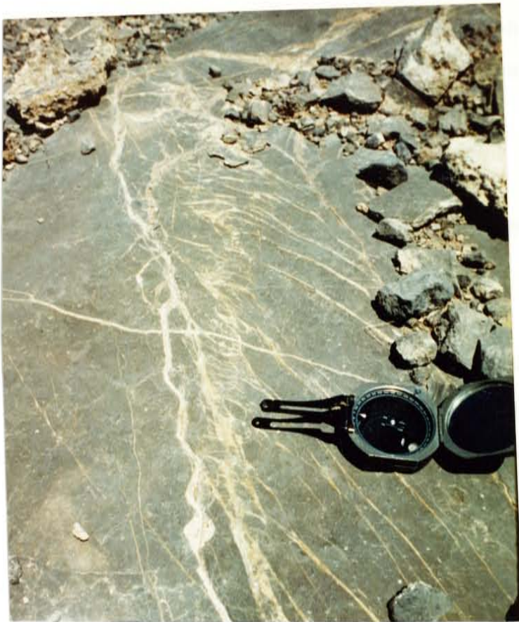
15: Moya Formation, right-stepping extensional fractures in s. 16.
