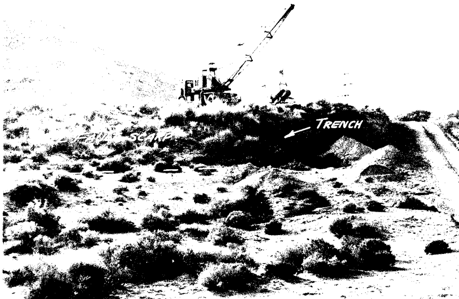
Dragline digging trench across the 1872 fault scarp at the north end of the Alabama Hills.
