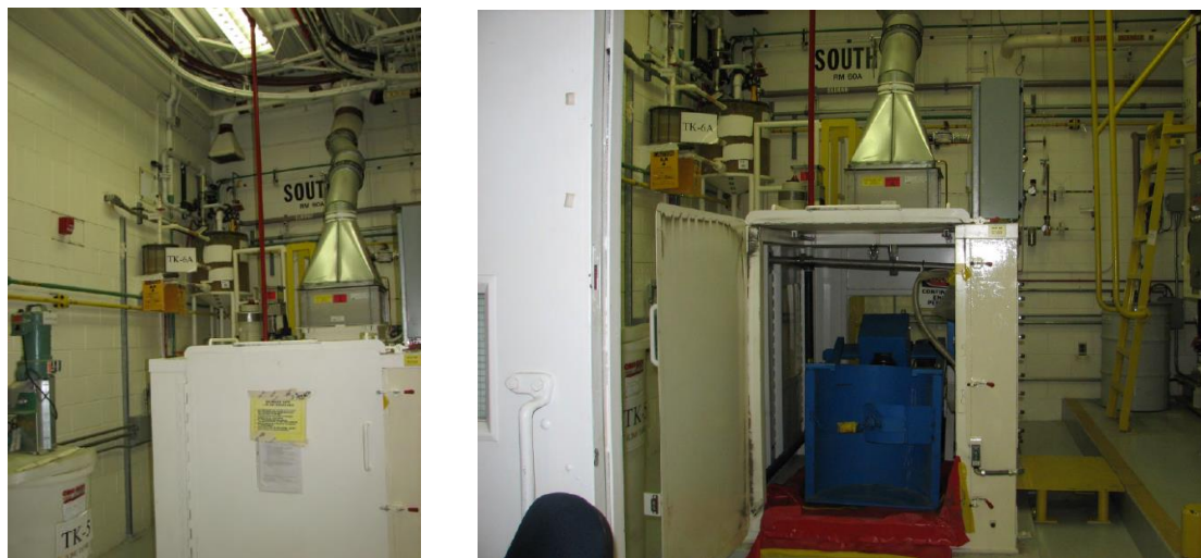
Figure 6 RLW drum tumbler and containment box
