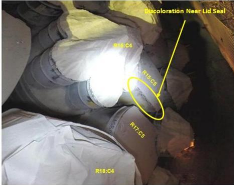
Figure 6-35: Discoloration of SWB at R15:C5
