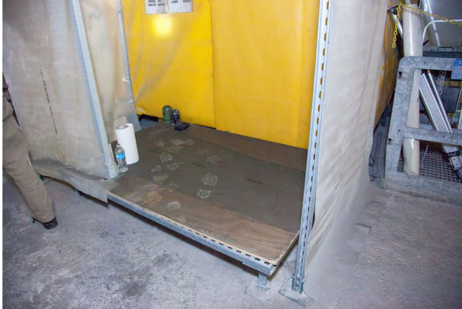
Figure 24: Soot Deposits in North Ventilation Circuit
