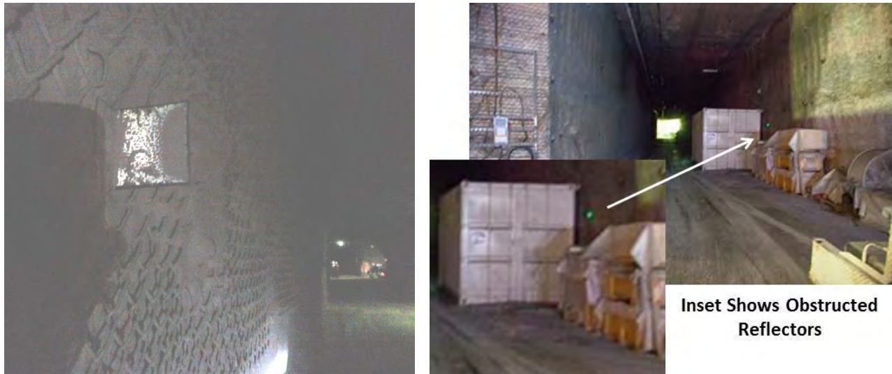
Figure 12: Obscured Reflectors
