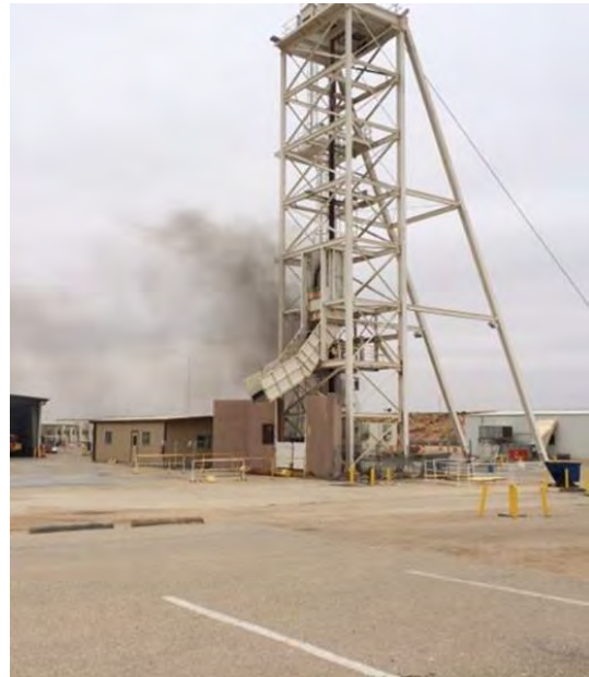
Figure 10: Smoke Visible Exiting through the Salt Shaft
