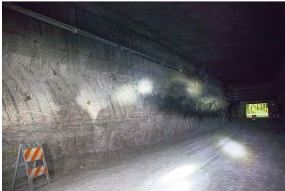
Figure 23: Smoke Signature on Rib (Looking South)
