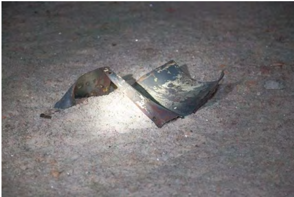
Figure 26: Damaged Access Plate
