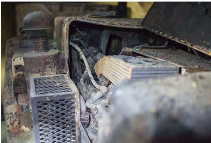
Figure 19: Engine Cooling Coils
