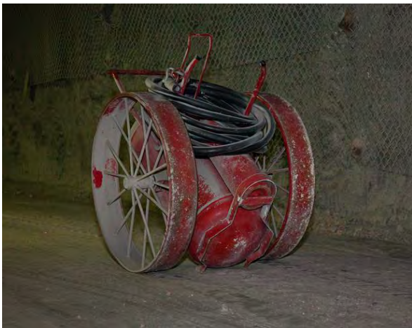
Figure 11: 300-Pound Extinguisher in the Underground
