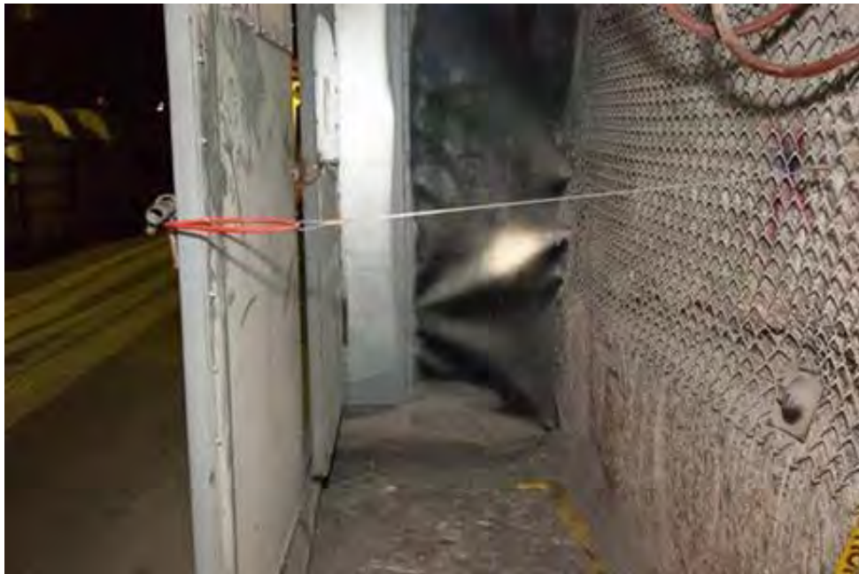
Figure 15: One of Chained Bulkhead Doors
