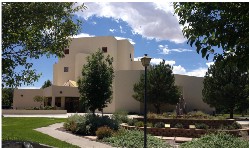
22 Workman Center, home of the Physics Department
