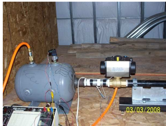
Figure 62: Reservoir, Ball Valve, Proto Board.
